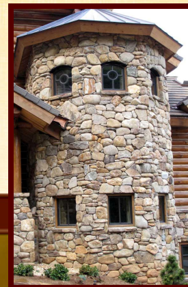
Stone Stair Tower
